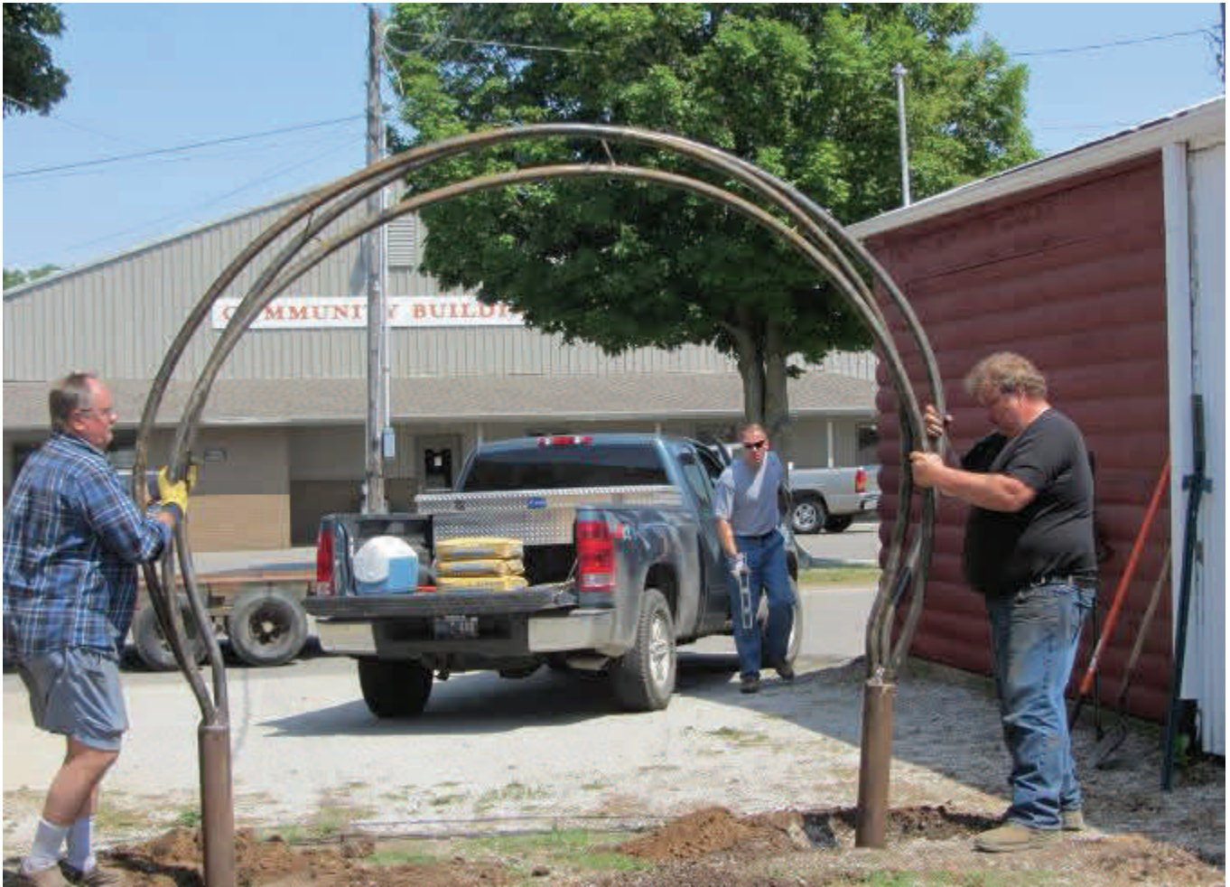
Hefting Arch into place
