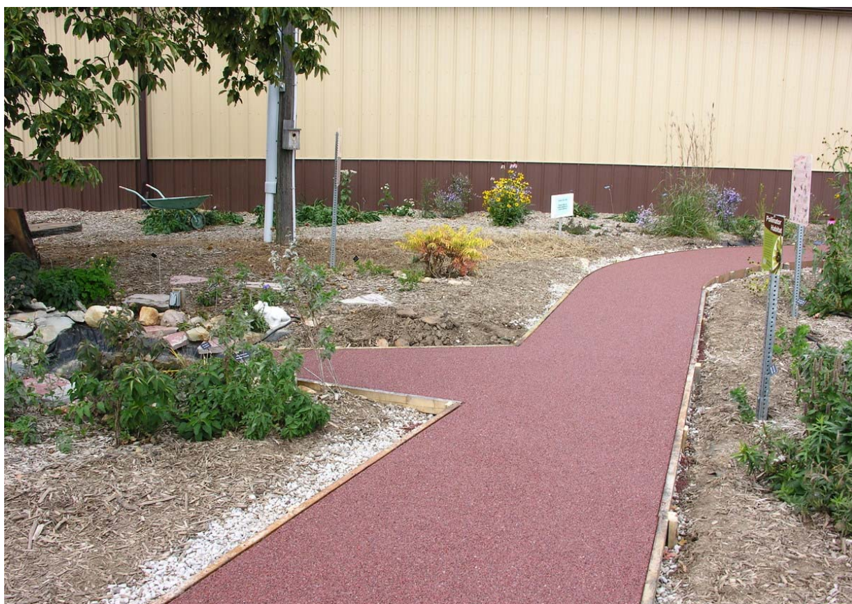
Beautiful new pervious FilterPave still in forms. Emerald Site Services custom-designed a portion so our spitting frog fountain demo drains back into the pond.
