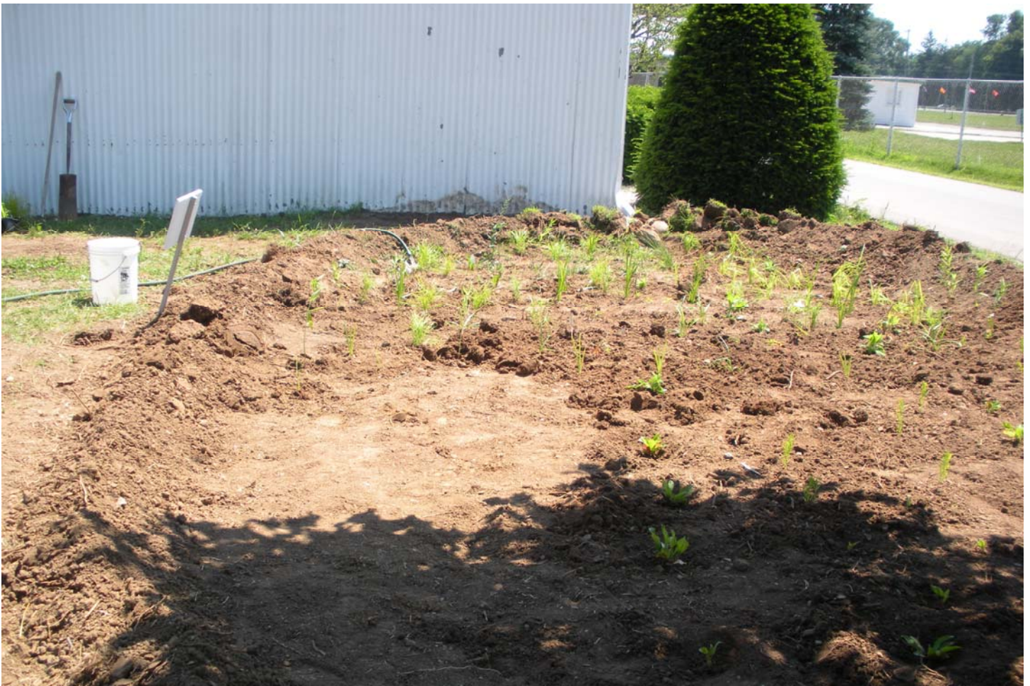
Raingarden after July 2011 workday. Outer 3/4 rototilled, larger earth berm established, additional plant plugs in place.
