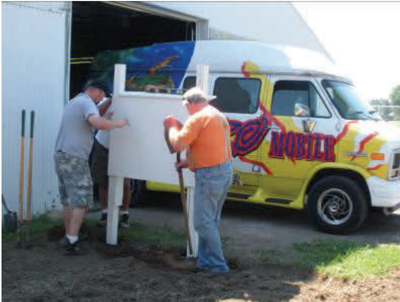
Installation of Kiosk sign
