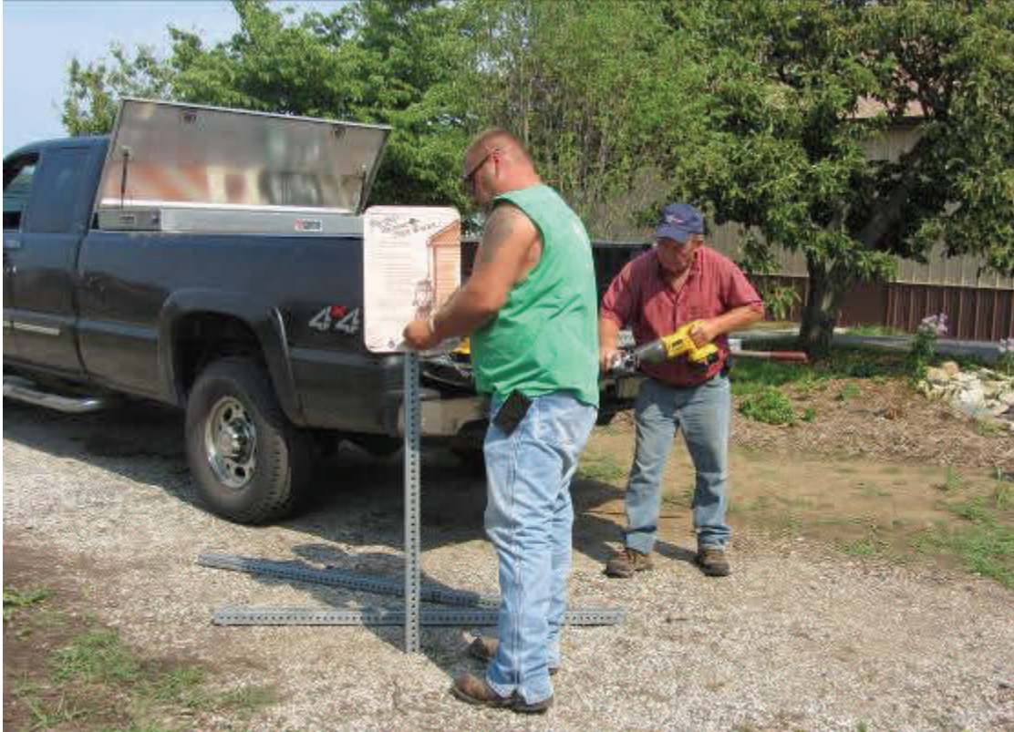
Partner Organization-La Porte County Highway installing signs
