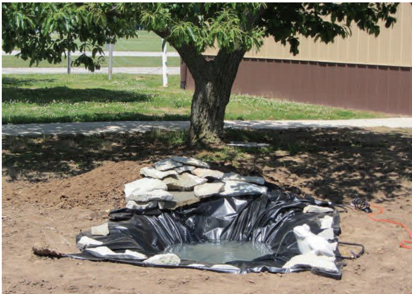
Liner in place & pump working
