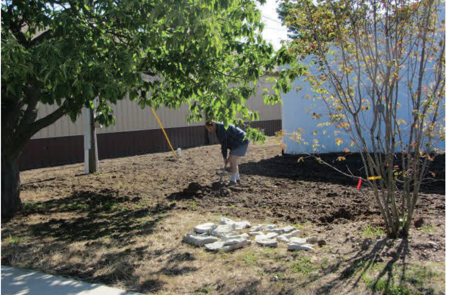
SWCD Supervisor Don Lode begins digging pond
